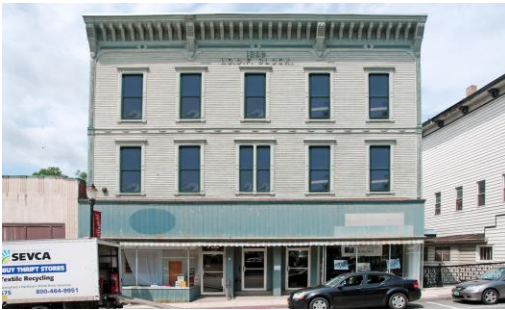
Figure 1 Odd Fellows Building - BEFORE
